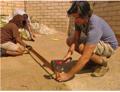
Prepare the Site
