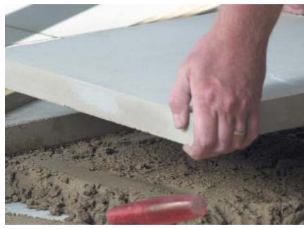
Begin the laying
