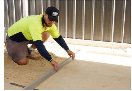
Level the surface
